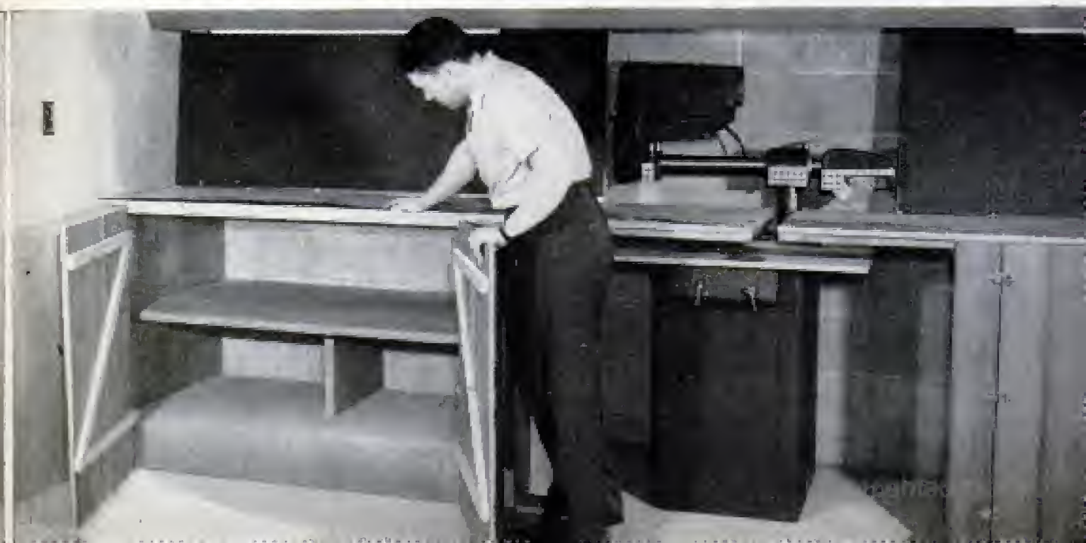
Simple cabinet construction can be seen from photo below. Note center shelf support and Z-bracing on doors
